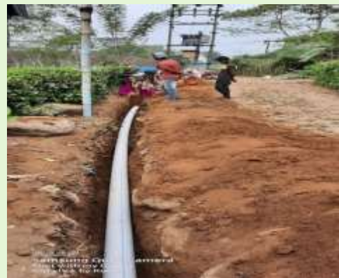
Earth filling on Pipe Line
